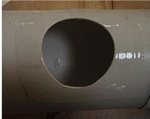
Figure 6 -- PVC Cement freshly applied to 4" Pipe
